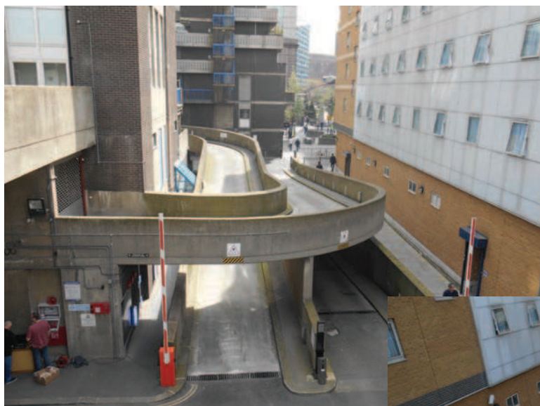
Photos of ramp before demolition Harrow Place end (August 2014)
